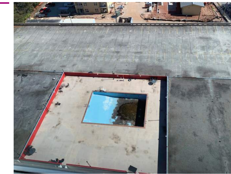
EXISTING PARKING LOT
