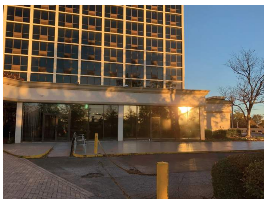
EXISTING STOREFRONT ON CAPITOL AVENUE
