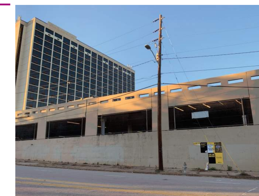
EXISTING PARKING LOT WALL
