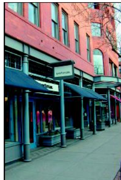
This building front also has variations in its depth. Steel columns define the building face at the sidewalk edge.
