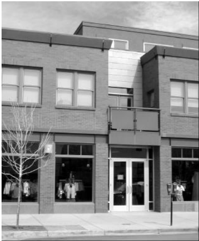
Architectural metal cladding used in limited amount
